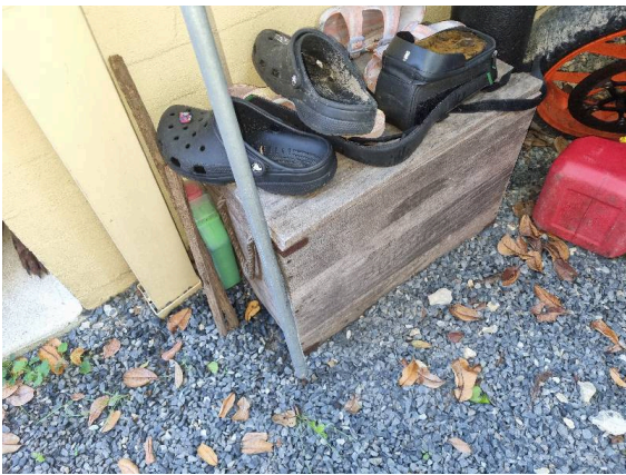
Example of stored timber in direct ground contact adjoining property which may attract termites. Unit 2.
